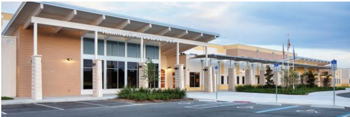
Photo Credit: Schenkel Shultz Architecture, Harmony Middle School Prototype
