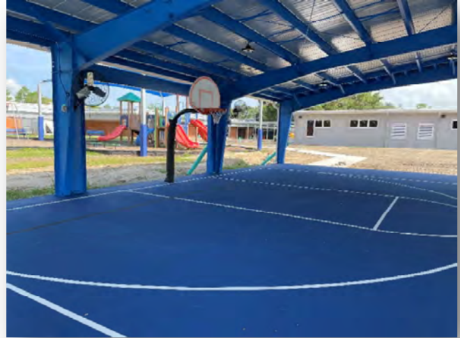
South Lake Elementary Covered Play, 2023 Photo Credit: BPS Facilities Services
