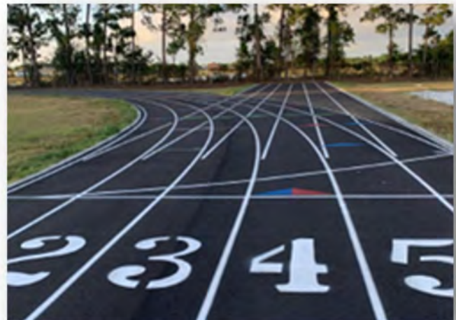
McNair Middle School Track Resurfacing Project, 2024 Photo Credit: BPS Facilities Services
