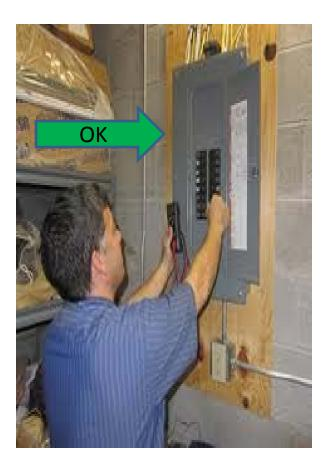
This is one type of a lock out tag out device used by a service technician when service is being performed
