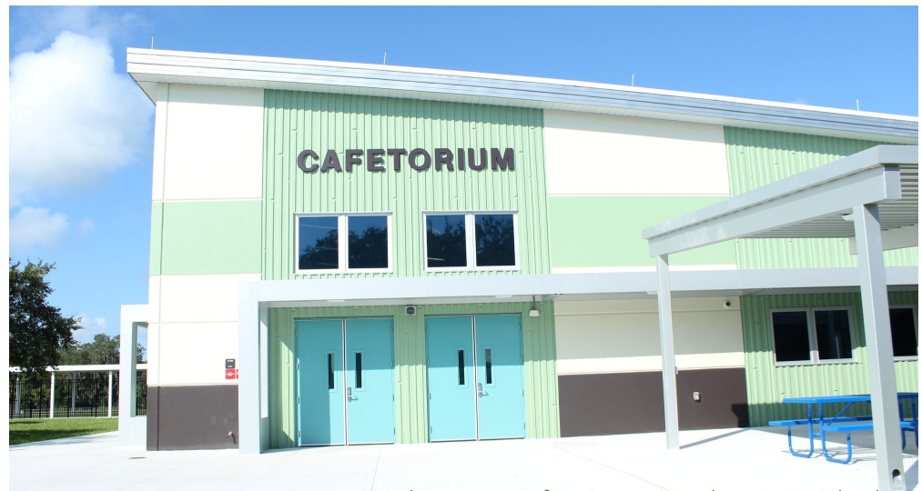
Photo: New Cafetorium, Mims Elementary School
