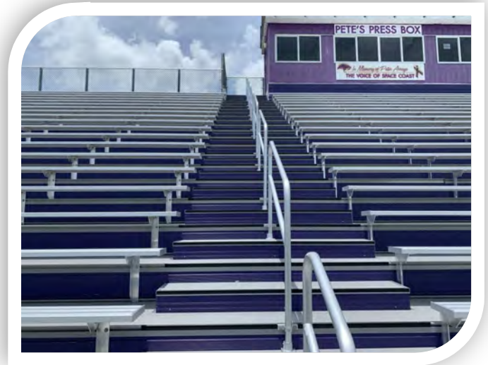
Space Coast Jr./Sr. High Grandstand Replacement, 2023
