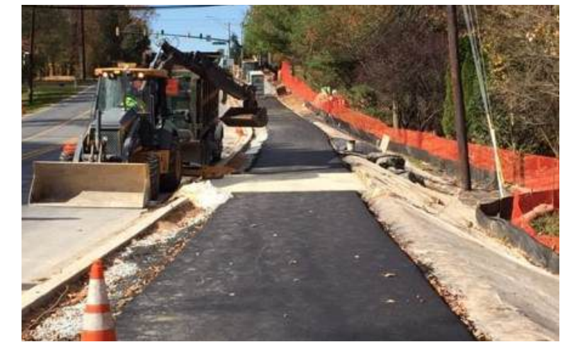
City trail under construction | Source: Montgomery County Government
