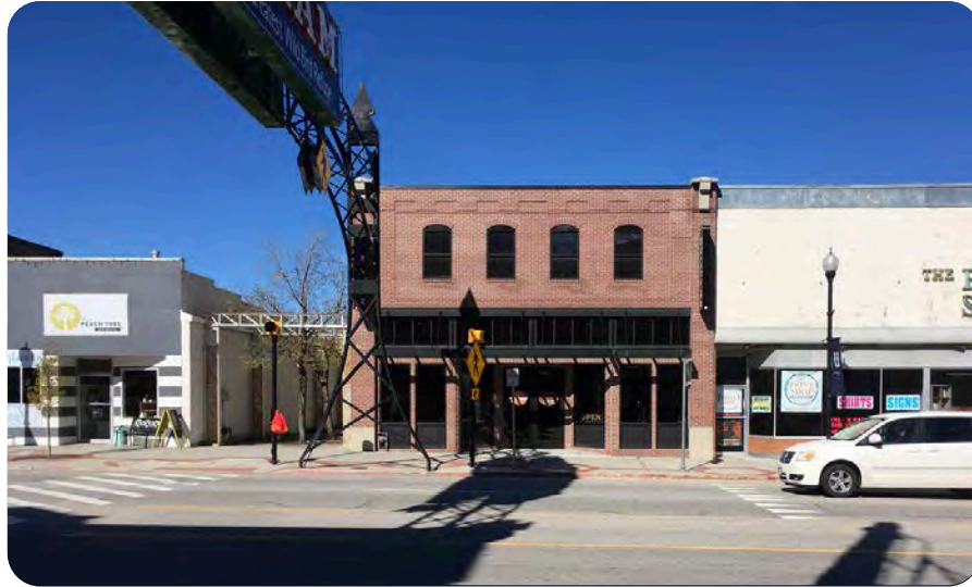
Recent building renovation on Main Street
