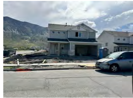
New Single-Family unit under construction in Brigham City
