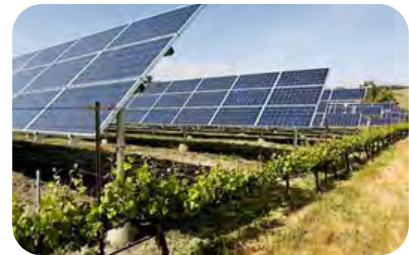
Small solar farm on Agricultural land | Source: Coldwell Solar
