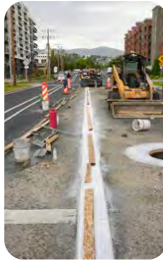
300 North road construction, Salt Lake City. Source: Salt Lake Tribune
