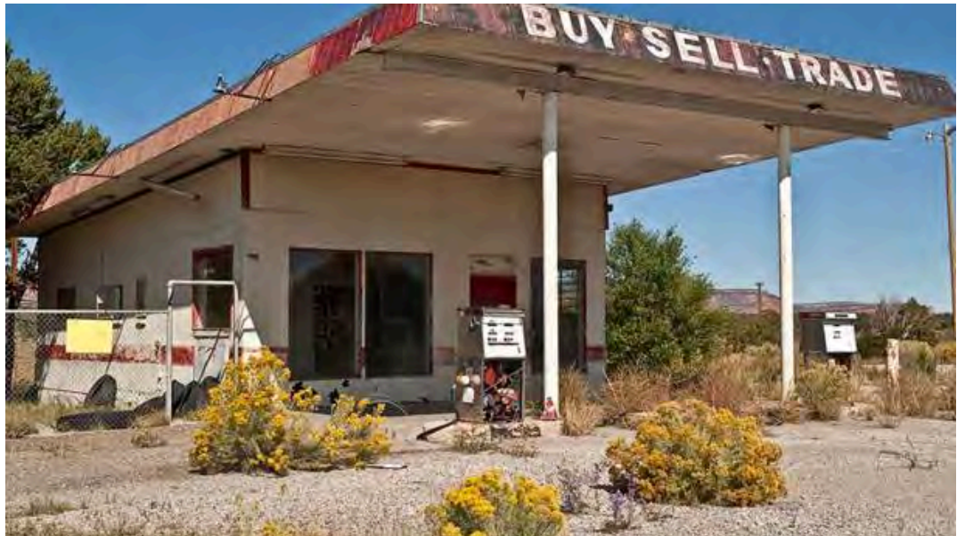
Example of brownfield site | Source: Choctaw Nation
