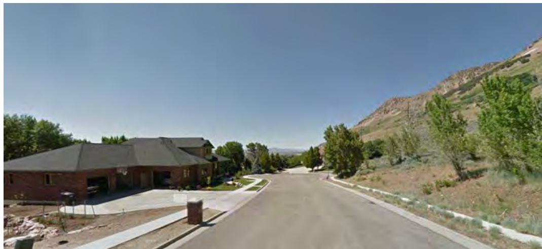
Upper hillside development on Marie Dr.
