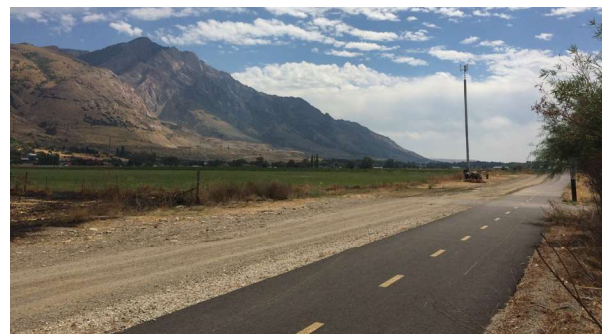
Figure 3-6. Existing section of the HOP located on the north end of Willard.
