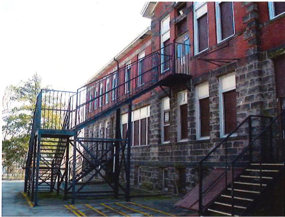
View of the rear (west) façade
