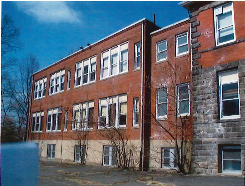
East façade of the southern most addition
