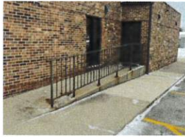
Rear Door Ramp
