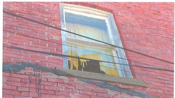
TYPICAL EXTERIOR FINISH CONDITIONS
