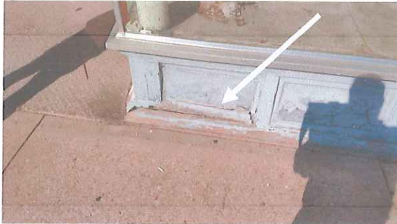
TYPICAL EXTERIOR FINISH CONDITIONS
