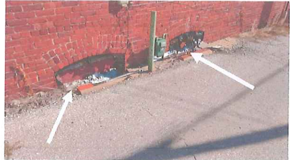
BASEMENT BACKFILL AGAINST ORIGINAL OPENINGS
