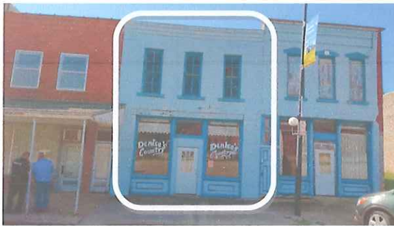
EASTERN STOREFRONT PORTION OF THE BUILDING
