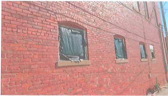
TYPICAL EXTERIOR FINISH CONDITIONS
