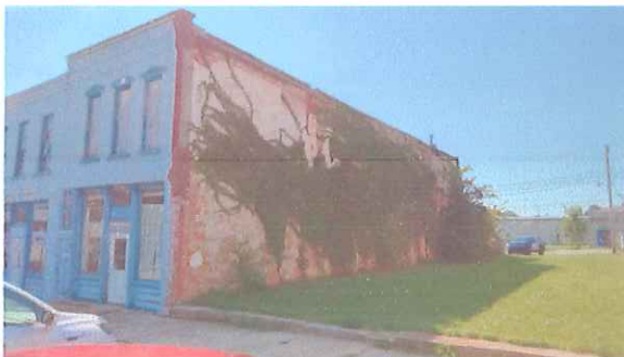
DEMOLISHED BUILDING'S SHARED WALL
