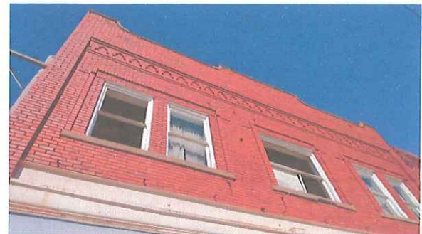
TYPICAL EXTERIOR FINISH CONDITIONS
