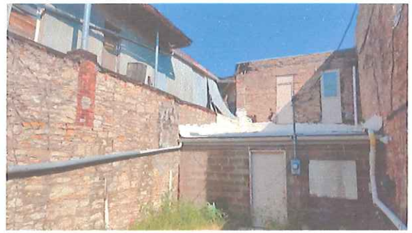
EAST BUILDING ELEVATION AT ADJACENT STRUCTURE
