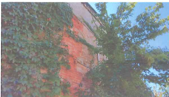
WESTERN WALL CONSTRUCTION MATERIALS
