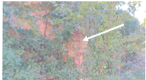
SOUTHERN WALL OF THE DEMOLISHED BUILDING
