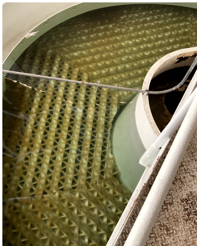
BOURBON RWD #4 TUBE SETTLERS
