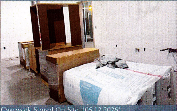
Casework Stored On Site (05.12.2026)
