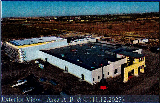
Exterior View - Area A, B, & C (11.12.2025)
