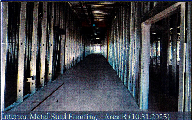
Interior Metal Stud Framing - Area B (10.31.2025)
