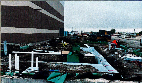
Plumbing Void System - Area F (04.09.2026)
