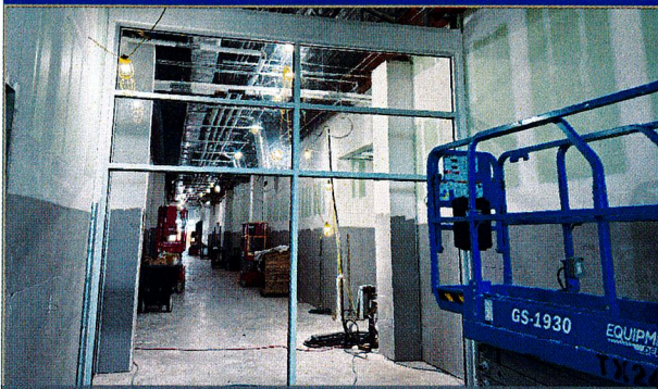
Interior Storefront Framing - Area A (04.02.2026)
