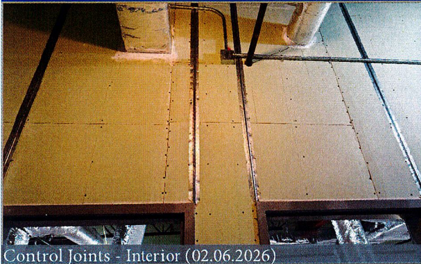
Control Joints - Interior (02.06.2026)
