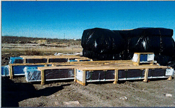
Exterior Finishes - Metal Panel (02.06.2026)
