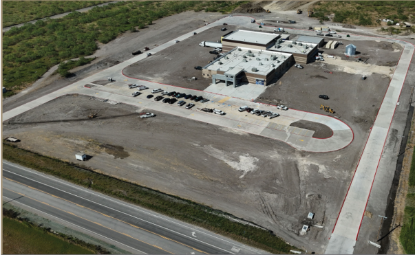
Site Paving - Concrete Drive (08.10.2026)
