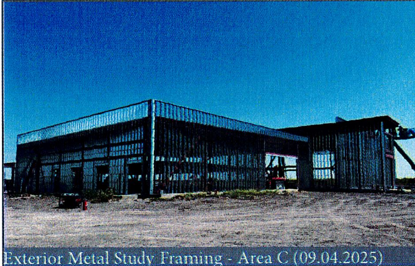
Exterior Metal Study Framing - Area C (09.04.2025)
