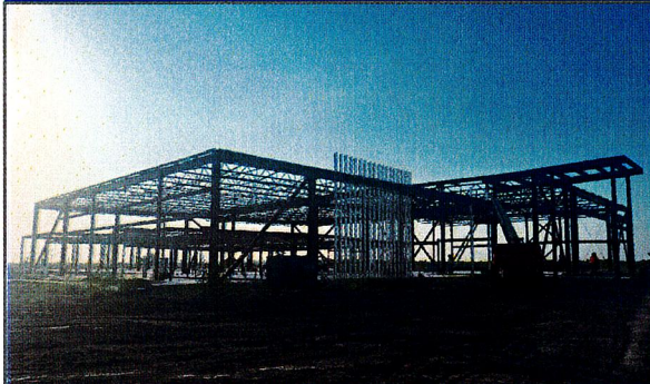
Exterior Metal Study Framing - Area C (08.07.2025)
