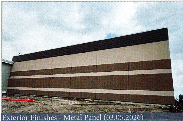
Exterior Finishes - Metal Panel (03.05.2026)
