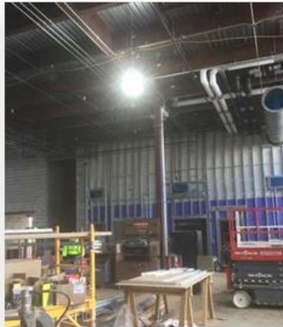
Continue MEP Rough-ins Area E
