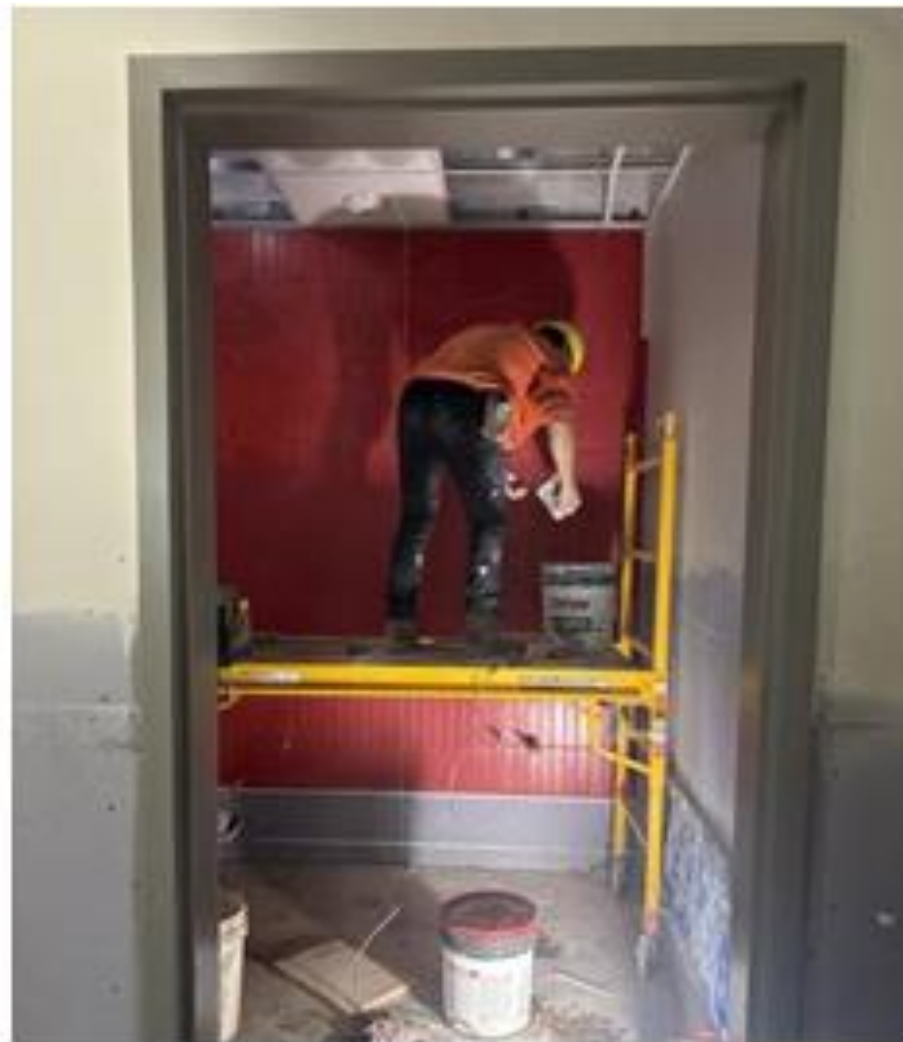
Red Tile Installation
