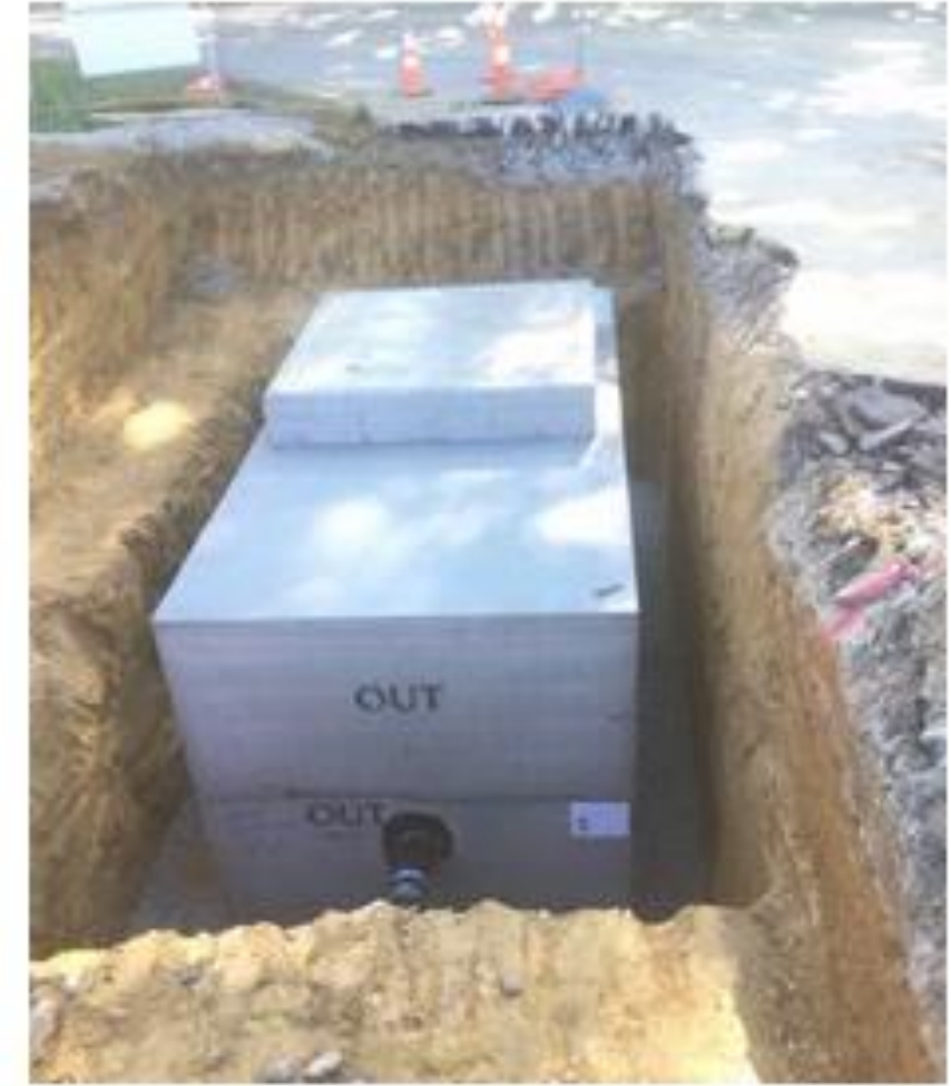
Water Meter Pit Installation
