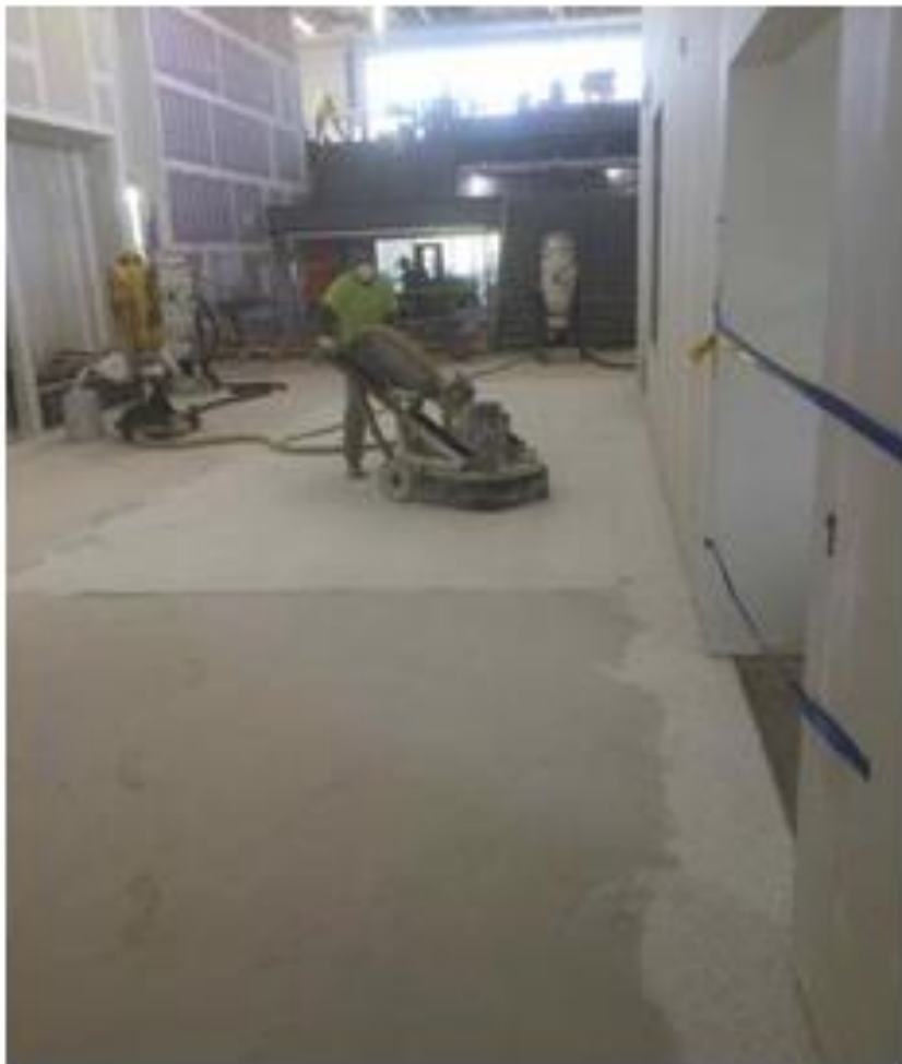
Terrazzo Grinding Main Entrance
