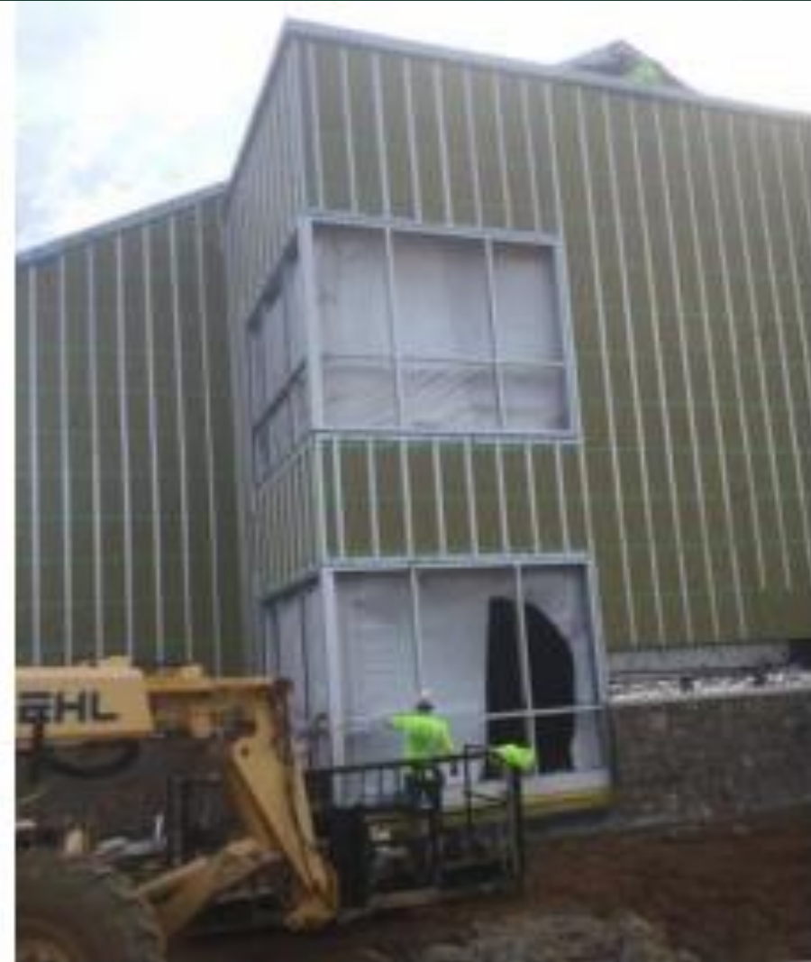
Aluminum Framing and Glazing Ongoing
