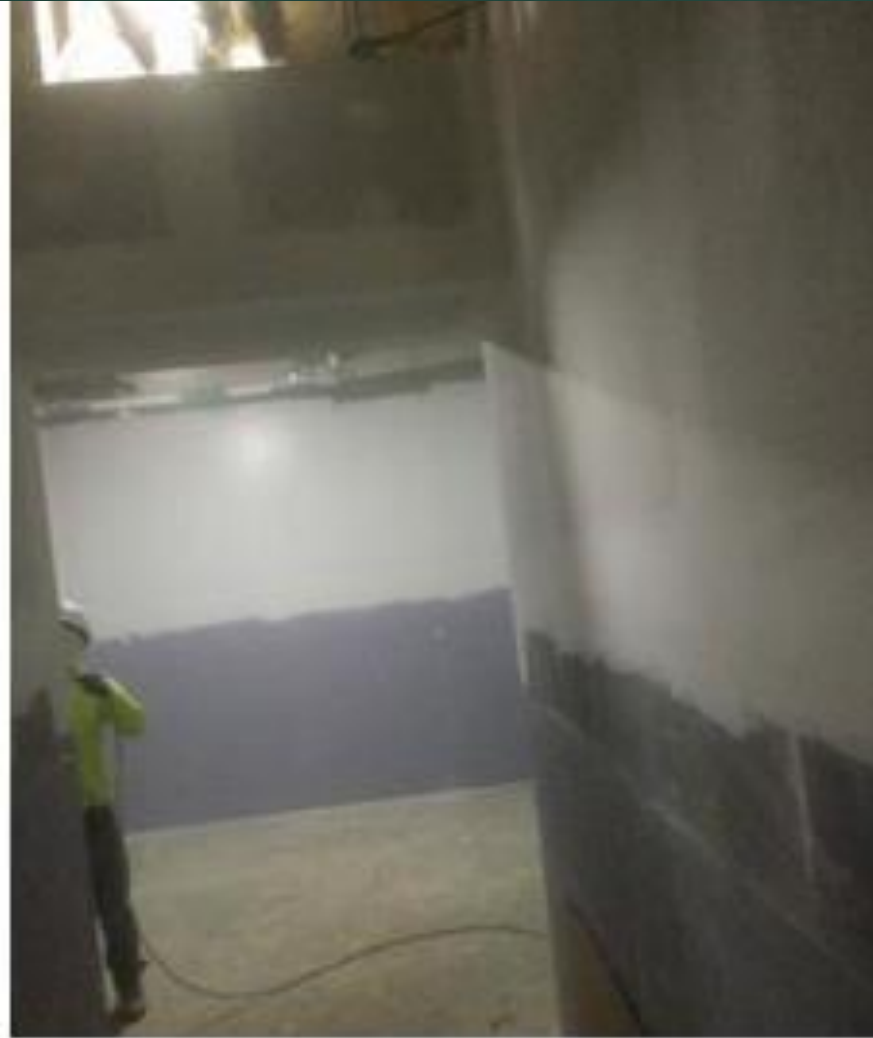
Beginning to Prime 1 st Floor Area A
