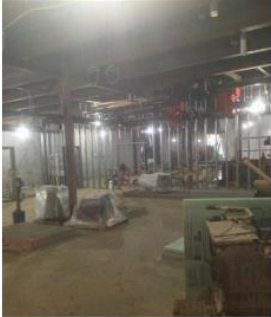
Framing and Mechanical Pipe in Area E
