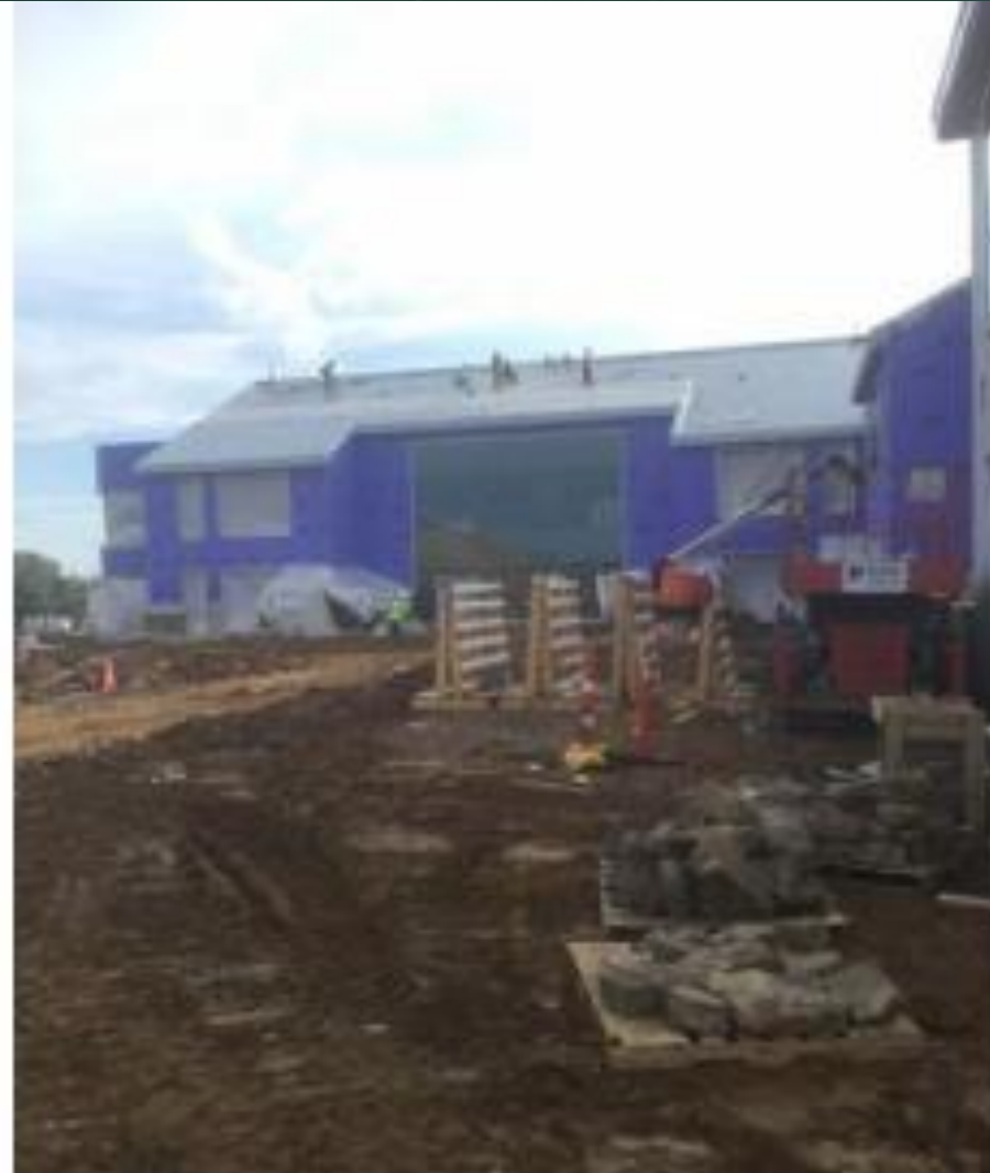
Sloped Roof Area D Continued
