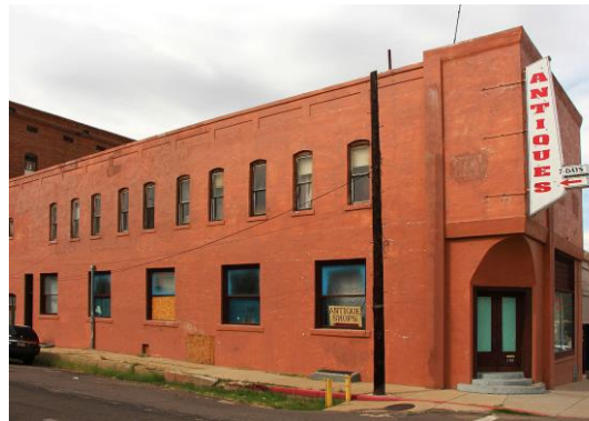
Butler Building - Eclectic
