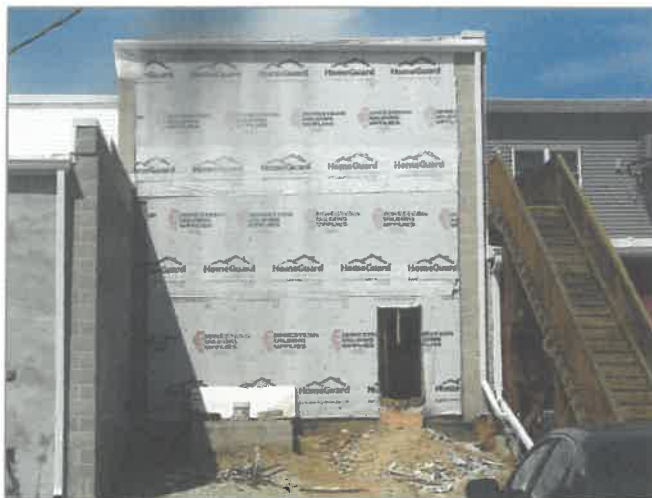
Figure 2. Rear, south-facing side of the building.
