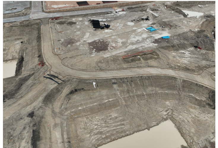
Start Forming Access Road #1
