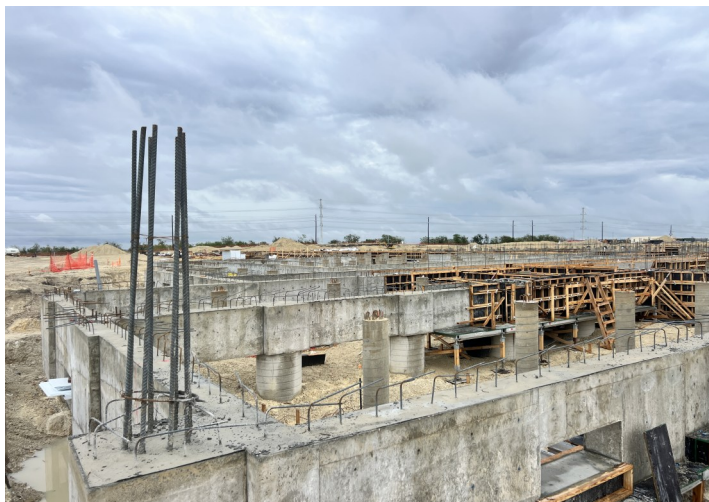
Place Grade Beams & Pier Caps - Area K
