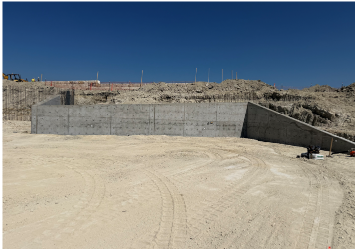
Cast In Place Retaining Wall #5
