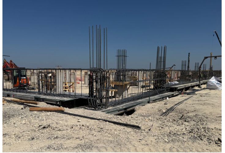
Area A Exterior Grade Beams
