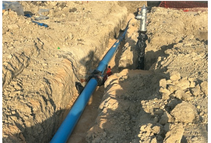
Install Fire Water Loop & Hydrant - Section 1
