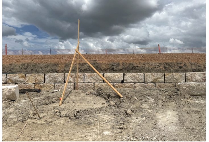
Begin Block Retaining Wall
