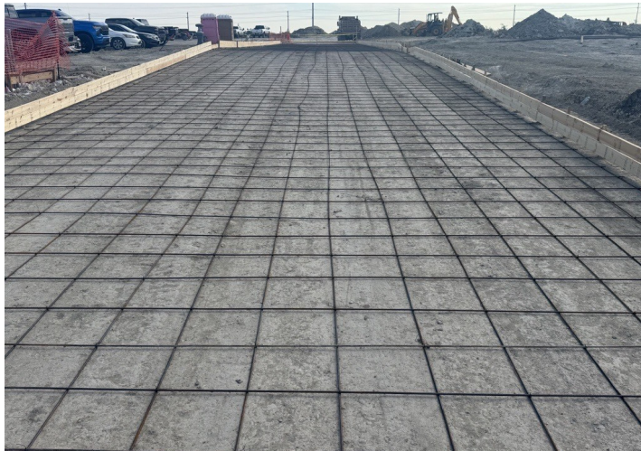
Form and Reinforce Section 2 Fire Lane Paving
