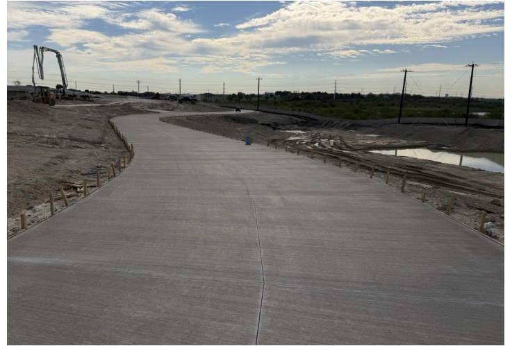
Access Road 1 Pavement
