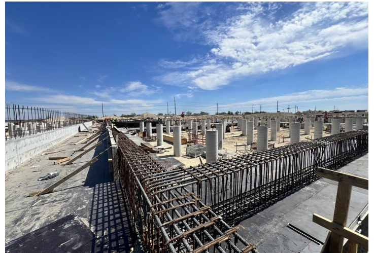
Grade Beam Reinforcing Area - N
