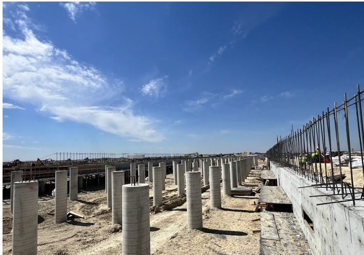
Place Grade Beams - Area L
