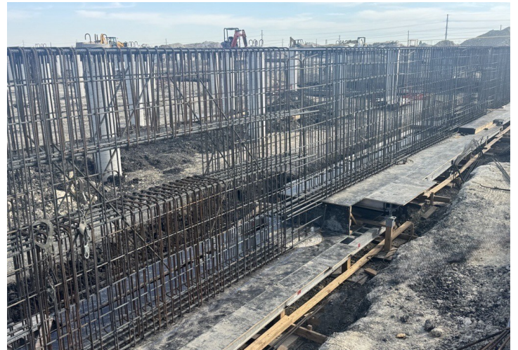
Form and Reinforce Area E Grade Beams
