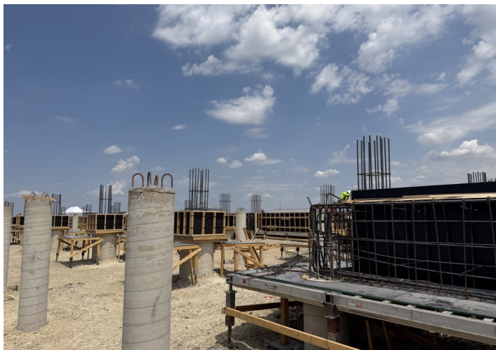
Areas A/B Rebar - Grade Beams & Pier Caps
