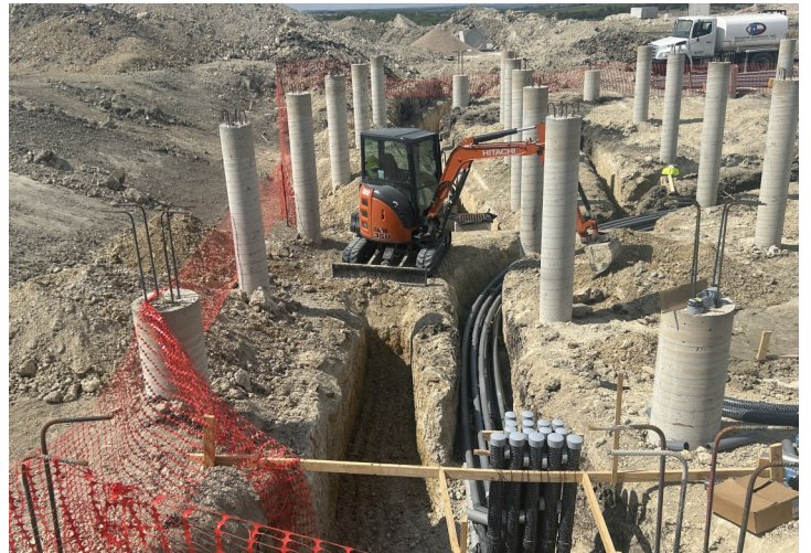
Area K - Electrical Underground
