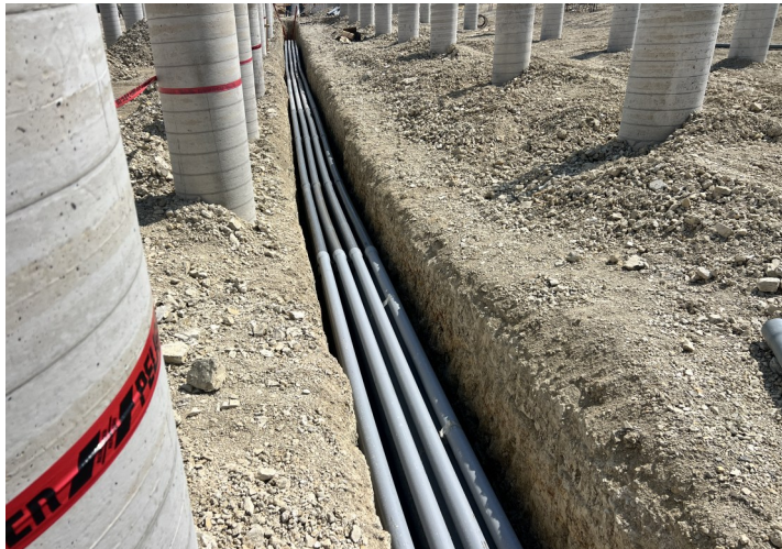
Area K - Electrical Underground
