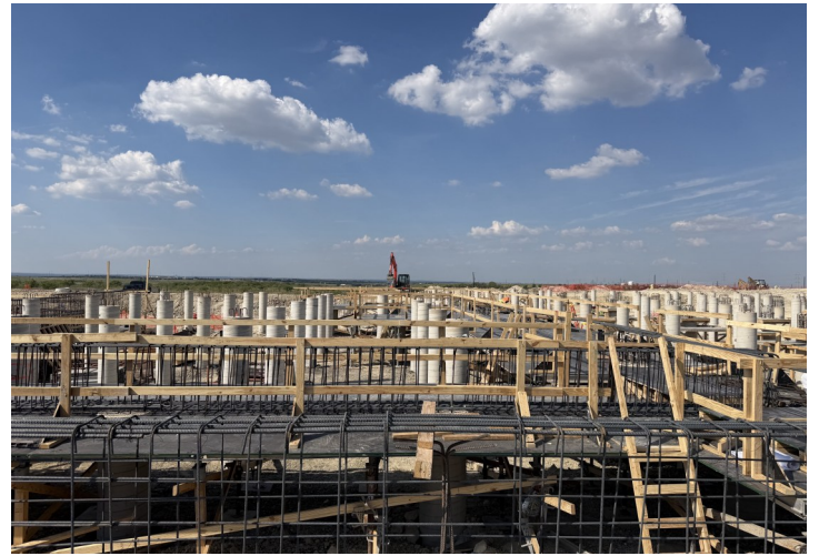
Forming Grade Beams & Pier Caps - Area E
