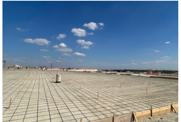
Forming & Rebar - Parking Lot 1
