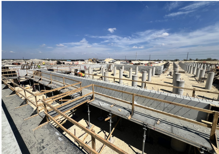
Place Grade Beams & Pier Caps - Area K
