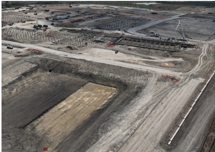
Continue Lime Stabilization & Fine Grade - Section 2
