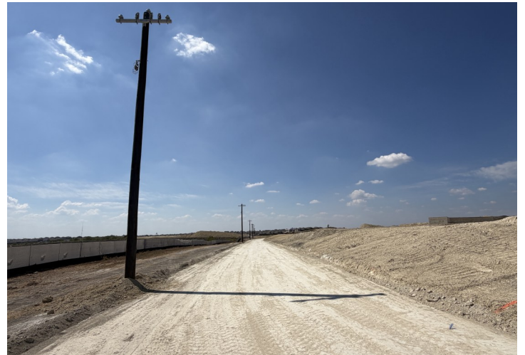
Install PEC Permanent Power Poles
