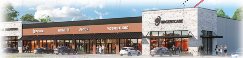
South Main Street Primary Commercial Corridor
