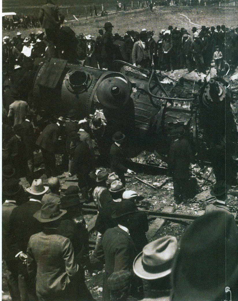
1901 Wildcat Engine. This is all that remained of one wildcat engine after five tons of dynamite exploded just east of the Vestal Depot.
