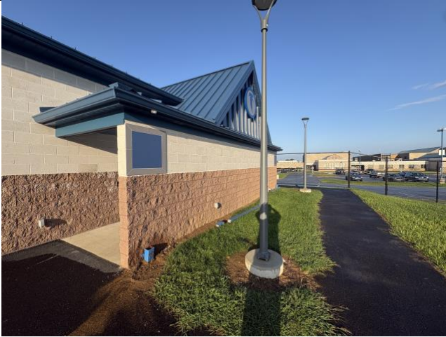
Exterior Tile on Both Fieldhouse Buildings
