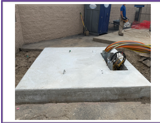
Transformer Pad Set
