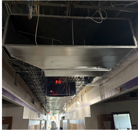
Duct Install Area A
