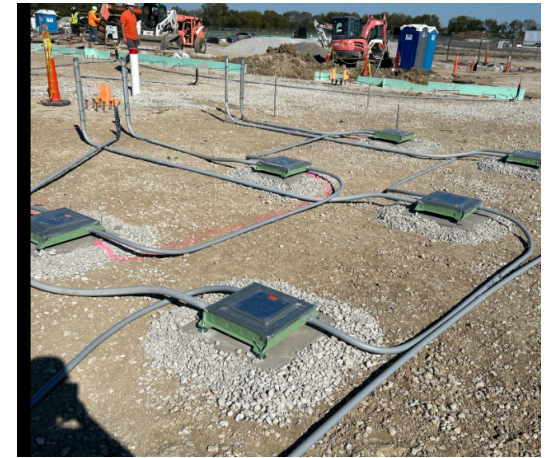
Floor Boxes Installed
