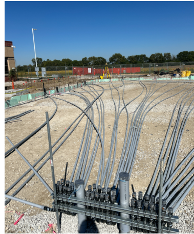
Underground Electrical Near Completion
