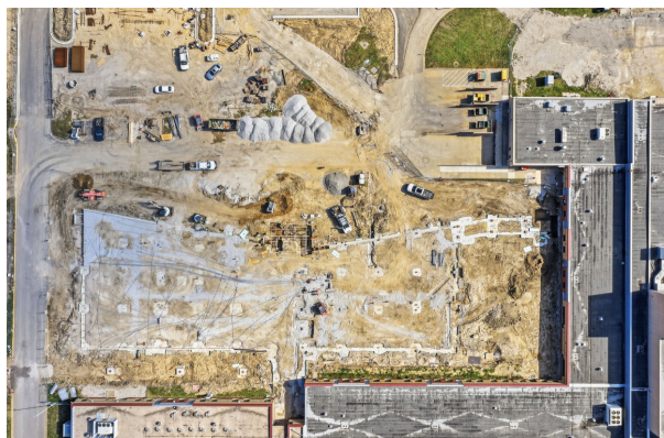
Drone Aerial Site View
