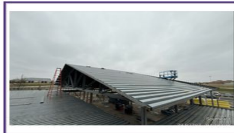
Decking Installed at Trusses and Flat roof
