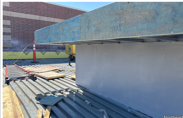
Soffit Fascia and Blocking
