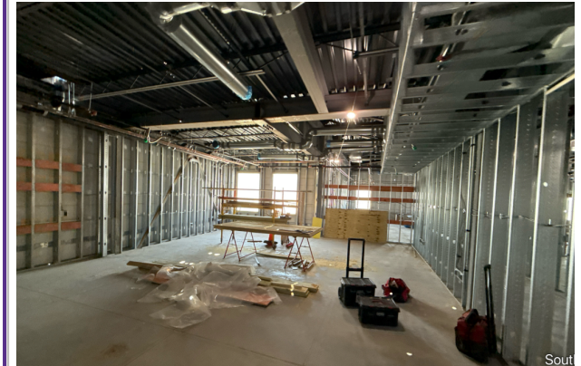
OH MEP Continues
