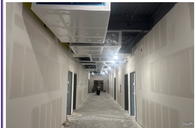
Drywall Finishing Continues
