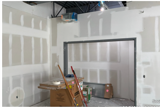
Finishing/Mudding Drywall
