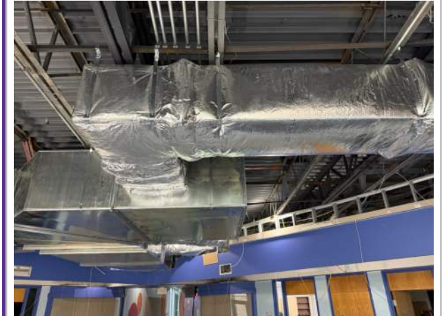
Duct installed in area B
