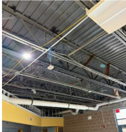
Joists have been installed
