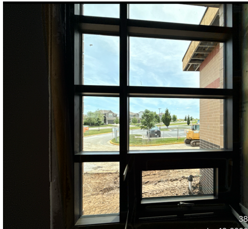
Glazing/ Glass installed
