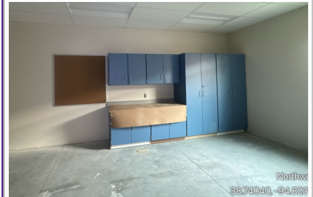
Marker/Tack Board Install + Casework Protected
