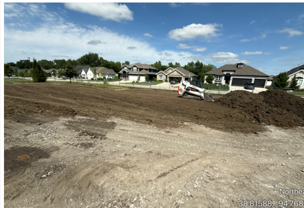
Laydown Yard Removed
