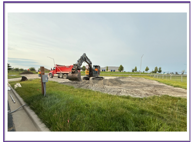
Laydown Yard Removed
