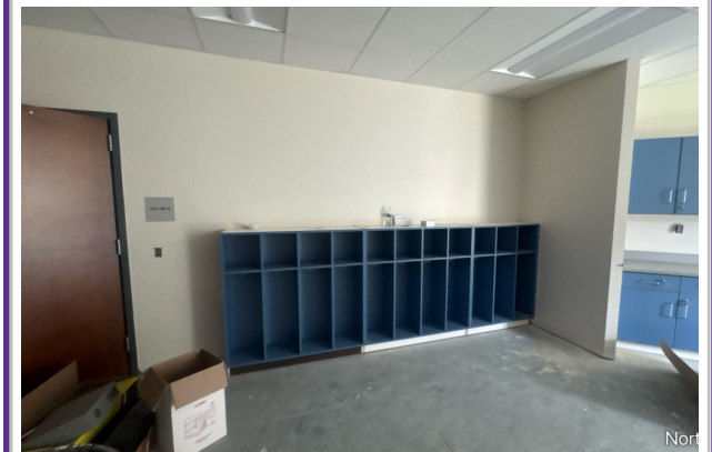
Tracking Remaining Casework (PLAM Tops)
