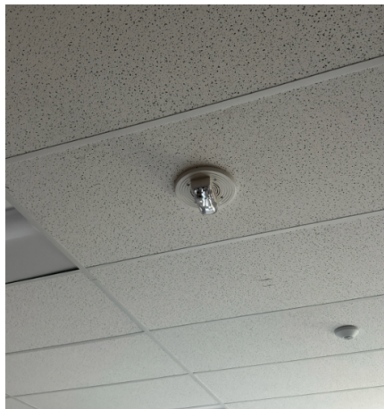
Remaining Low Voltage Device Install
