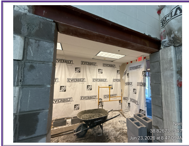
PCE Office - New Door Opening/ Lintel for frame
