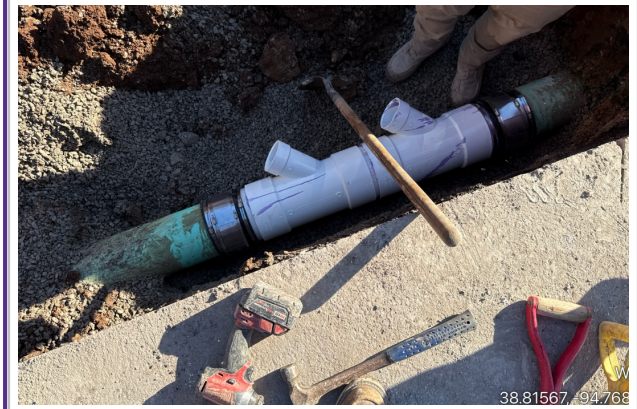
Utility Tie In
