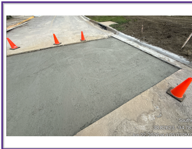
Road Work for Asphalt Patch Back (lay base)
