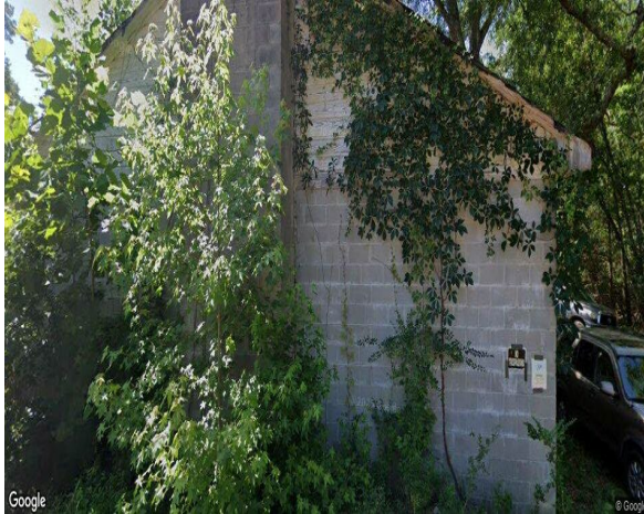
114 Scout Circle – vacant outbuilding- Zoned 501
