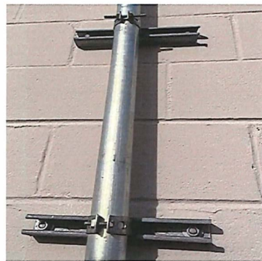
Wall Mount Sections with Hinged Base and Hardware
