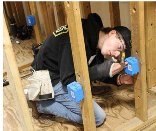
Student works on electrical framing project during SkillsUSA competition.
