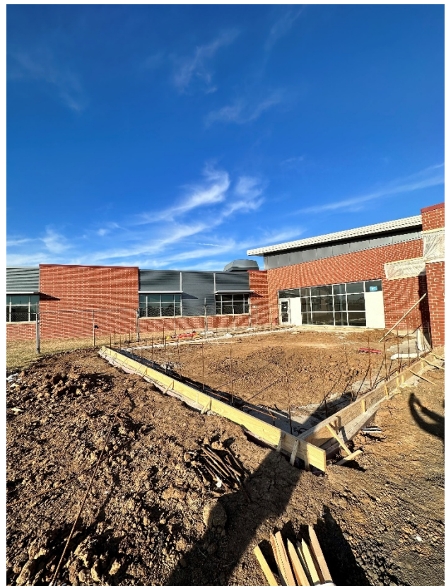
Cafeteria slab on grade forms complete (November 14, 2023)
