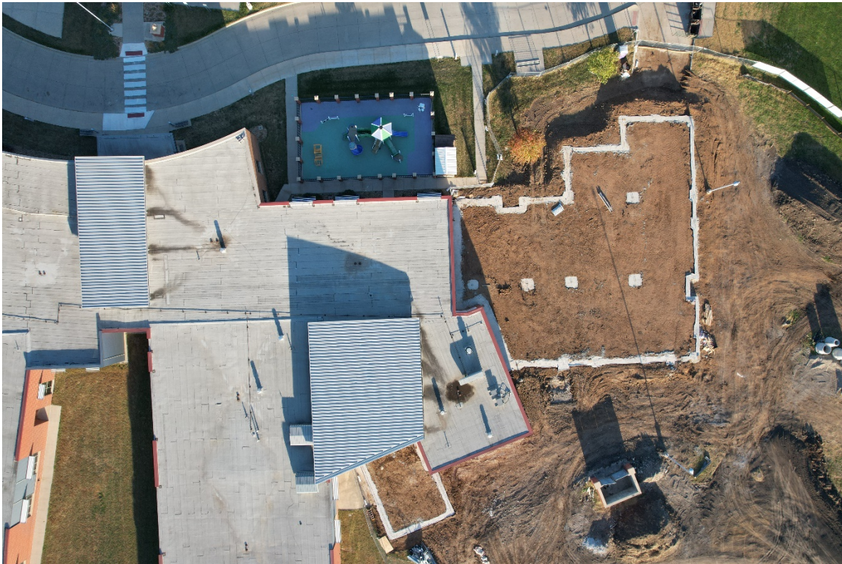
Concrete footings complete (October 17, 2023)
