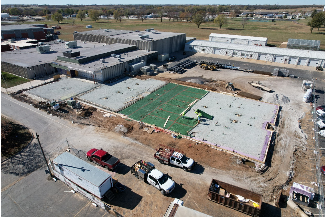
Slab on grade vapor barrier in progress. (October 31, 2023)
