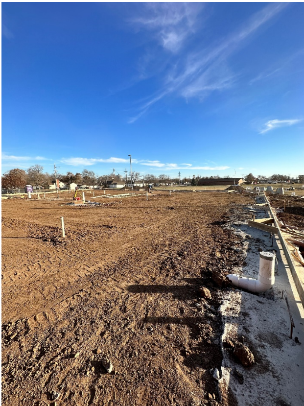
Slab on grade forms complete (November 14, 2023)
