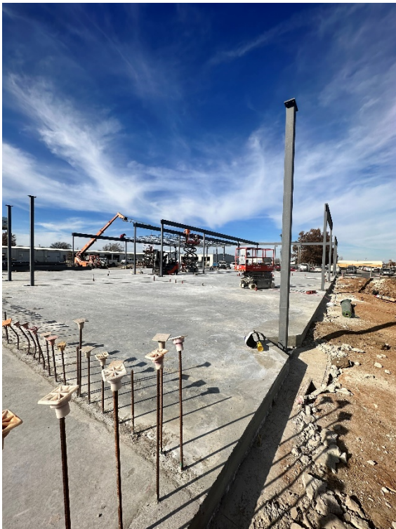
Steel erection in progress (November 14, 2023)
