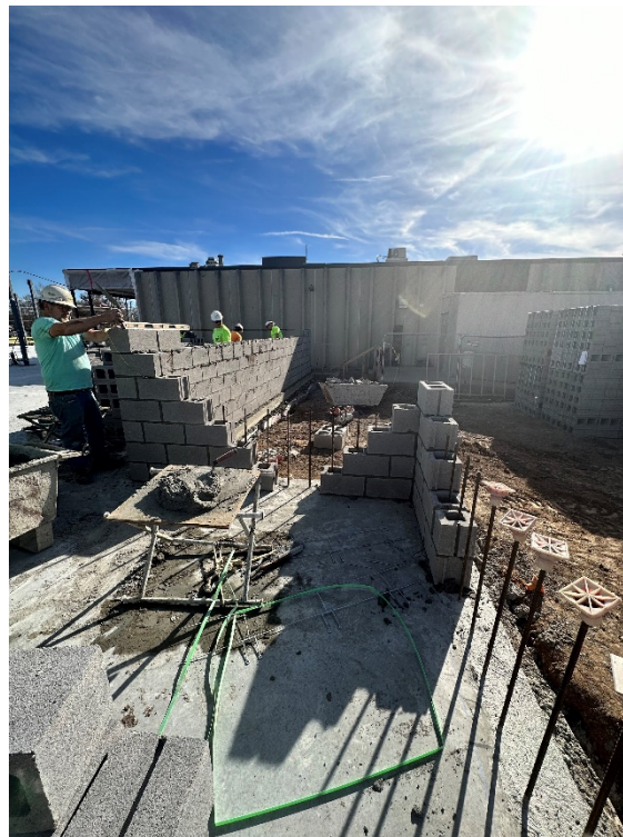
Masonry installation in progress (November 14, 2023)
