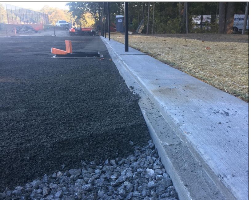
FIELD EDGE AND BASE CONCRETE TURF ANCHOR CURB WITH INTEGRAL FENCE POSTS. 8" STONE BASE WITH 2" TOPPING STONE AND 6" DYNAMIC STONE BASE. SIEVE AND LA ABRASION TESTING TO MEET FIELDTURF STANDARDS
