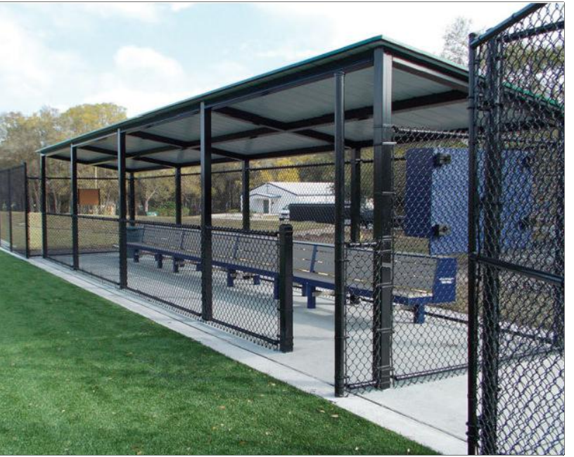
DUGOUT SHADE STRUCTURE SHADE STRUCTURE DUGOUT ON CONCRETE BASE WITH FENCE SURROUND
