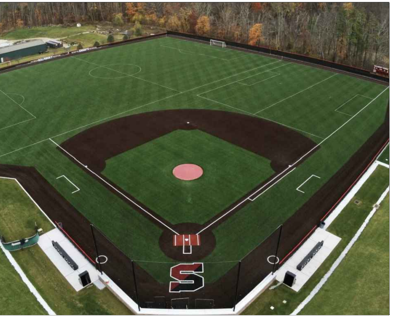
BACKSTOP AND HOME PLATE LOGO ALL BACKSTOPS TO BE 30' HT. TENSION NETTING ABOVE 6' HT. HEAVY DUTY FENCING. 24' TALL NETTING ABOVE FENCE. AS MANUFACTURED BY SPORTSFIELD SPECIALTIES OR JAYPRO SPORTS
