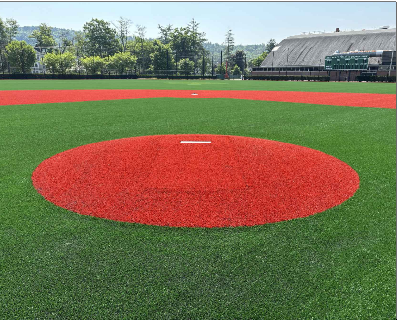
EASY CHANGE MOUND FIELDTURF EASY CHANGE MOUND SYSTEM FOR GAME FIELD. REPLACEABLE SECTIONS OF MOUND SET IN CONCRETE PAN FOR EASE OF REPLACEMENT. 3 REPLACEMENT SETS INCLUDED
