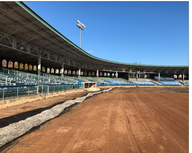
SUBGRADE WITH COLLECTOR PIPE LASER GRADE AND PROOF ROLL SUBGRADE. PITCH TO COLLECTOR PIPE AT LOW POINT. INSTALL 8"-12" COLLECTOR PIPE AND OUTLET.
