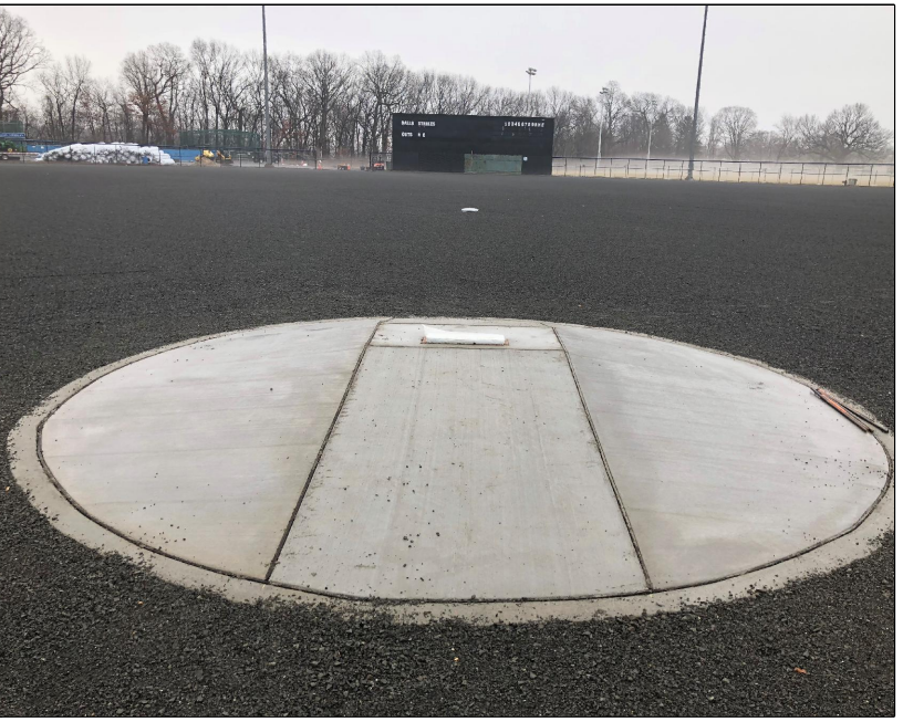
PITCHING MOUND CONCRETE MOUND FOR STABILITY AND LONGEVITY FOR GAME MOUND
