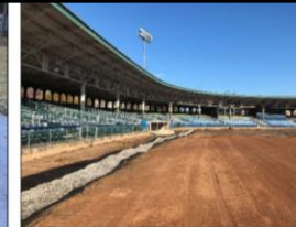
SUBGRADE WITH COLLECTOR PIPE
