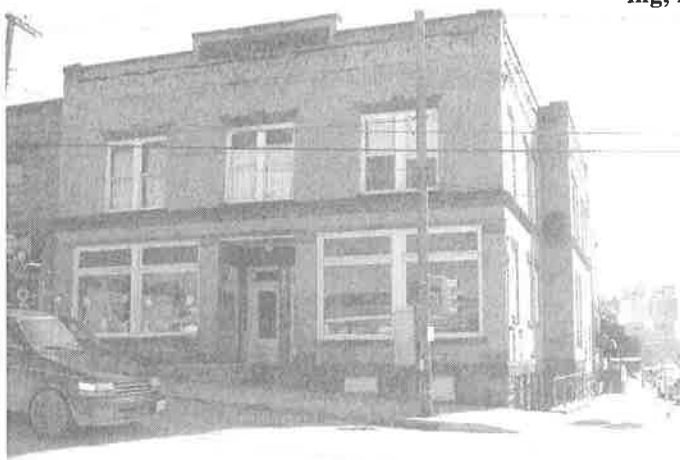
The Clymer National Bank building as it appears today. Photo by Brian Church.
