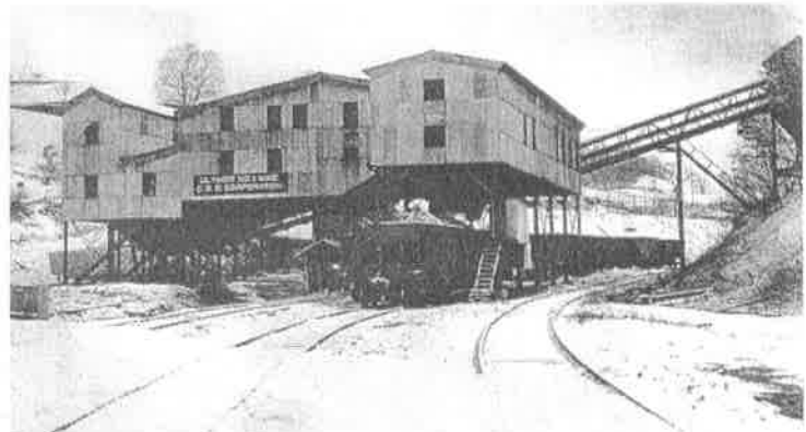
The mining tippie used by the CBC for mine number one. Photo courtesy of John F. Busovicki.
