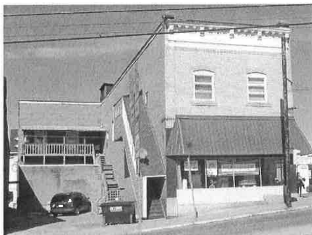
The Clymer Hardware building as it appears today. Photo by Brian Church.
