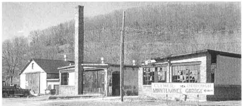
Current picture of the CBC Machine storage and repair building, it is now owned by Clymer borough. Photo by Brian Church.
