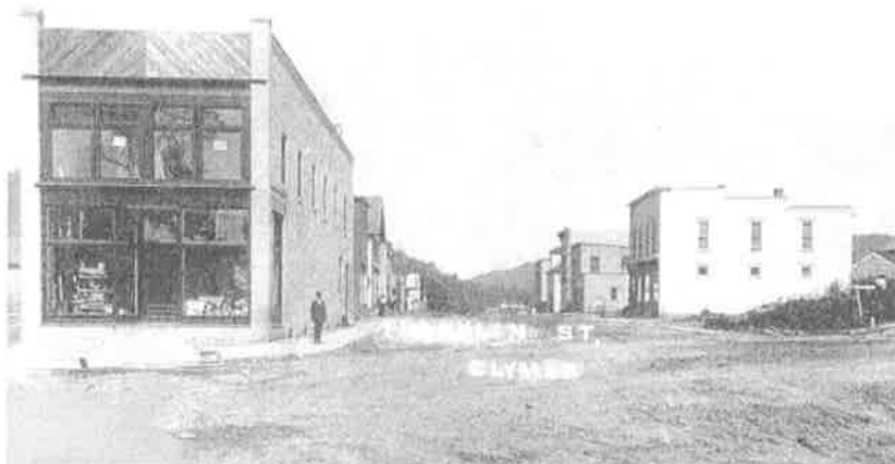
Newly constructed Clymer Hardware store 1907. Photo courtesy of John F. Busovicki.
